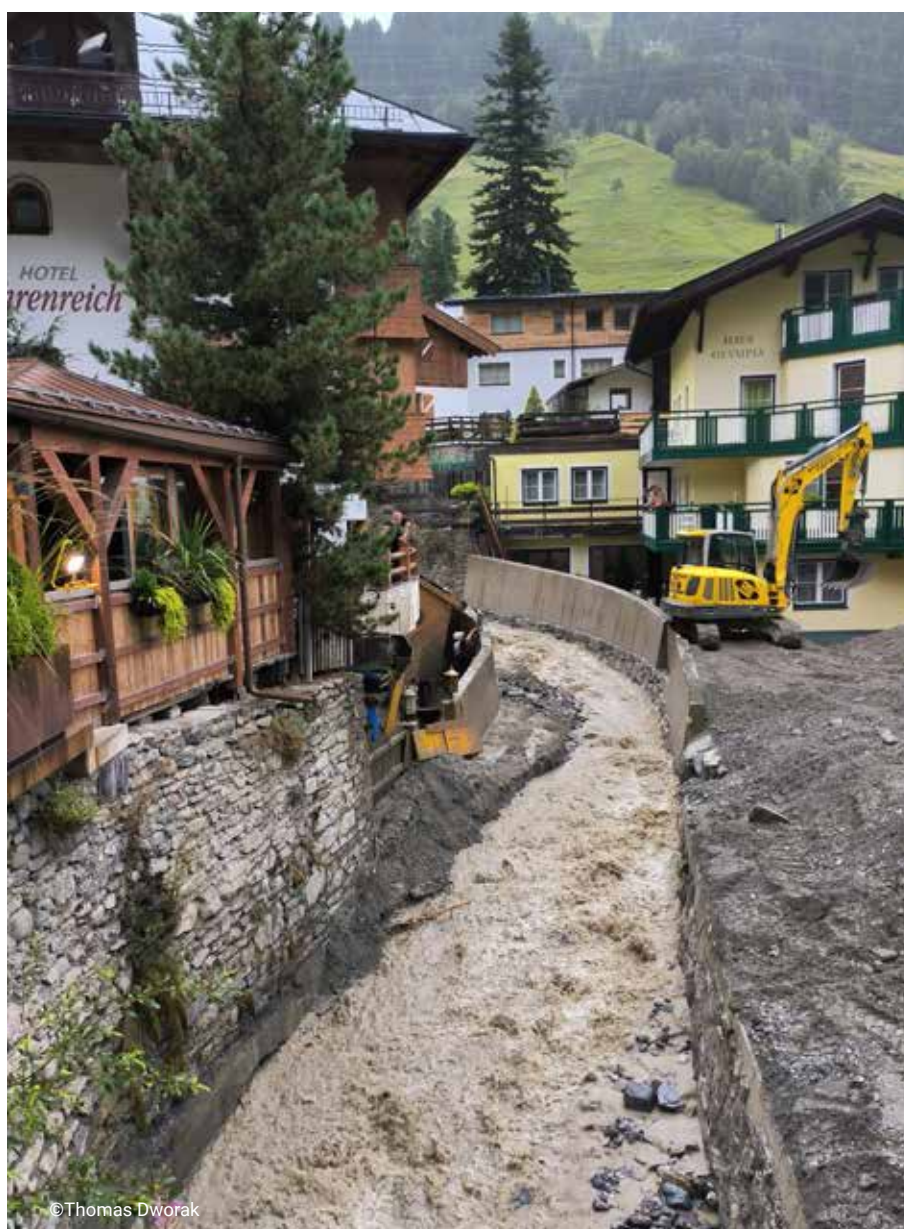
Figure 4.5 Impact of a flash flood in Austria, summer 2024
