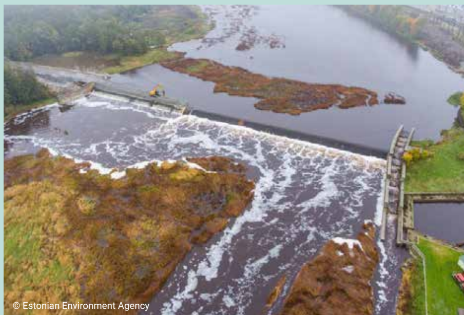
Figure 2.7 Aerial view of the Sindi Dam before removal
