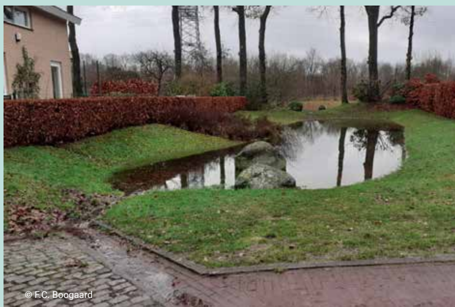
Figure 4.6 Swale in a housing area
